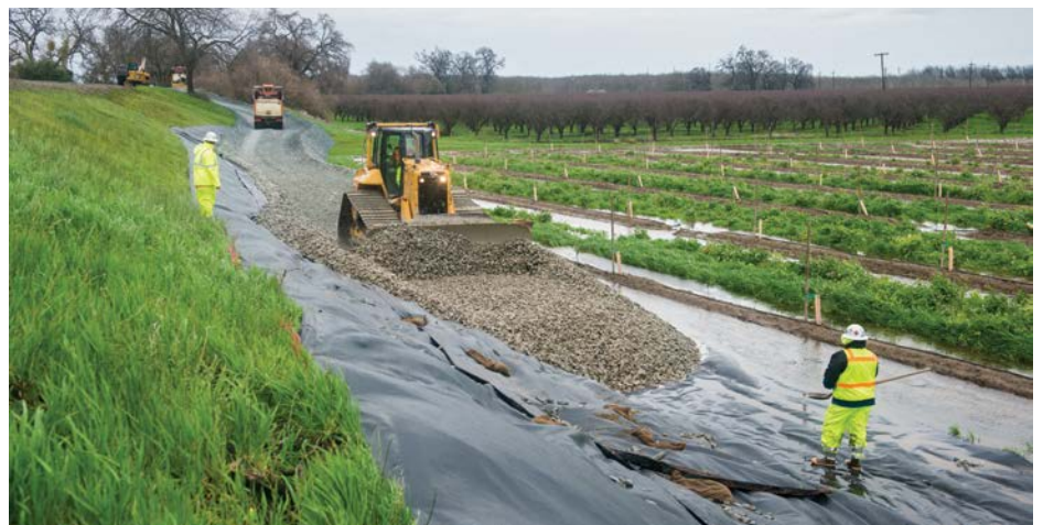
A Delta levee being repaired.
