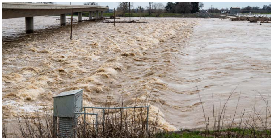
Flooding on the Sacramento River in 2019 overtopped the Tisdale Weir.
