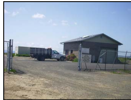
Wastewater Treatment Facilities
