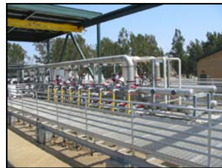
American Canyon WWTP
