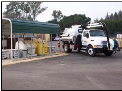
Wastewater Treatment Plant
