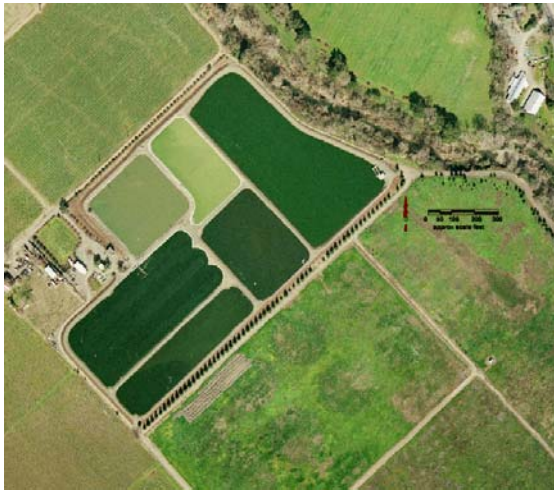
St. Helena WWTP
