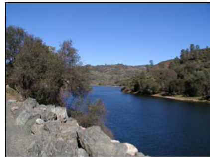
Putah Creek Intake
